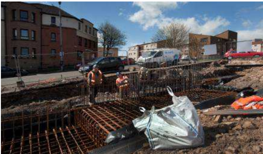
On site at Maryhill Health and Care Centre
