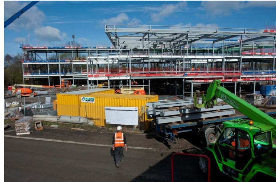
On site at Eastwood Health and Care Centre
